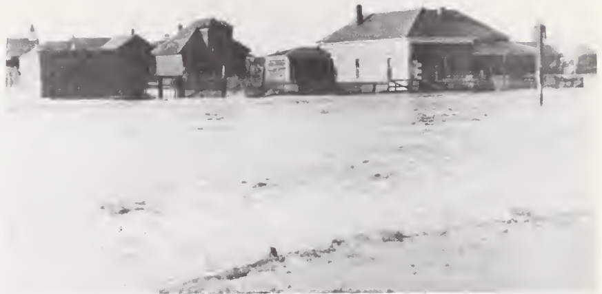
Floodwater damage to urban property in Van Horn from the flood of September 4, 1913. This flooding was prior to the railroad constructing a diversion around the city of Van Horn.
